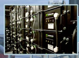
The liquid-cooled batteries are stored in two seperate rooms, each room holds 420 battery modules.
